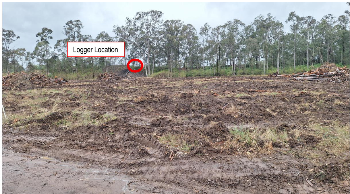
Figure 5: In-situ logger location, far view –standing onsite and facing south (1/7/25)
